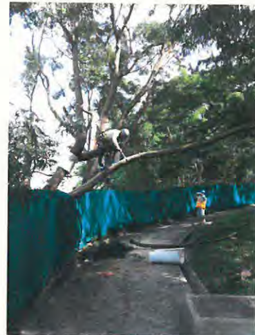
Tree Climbing for pruning works
