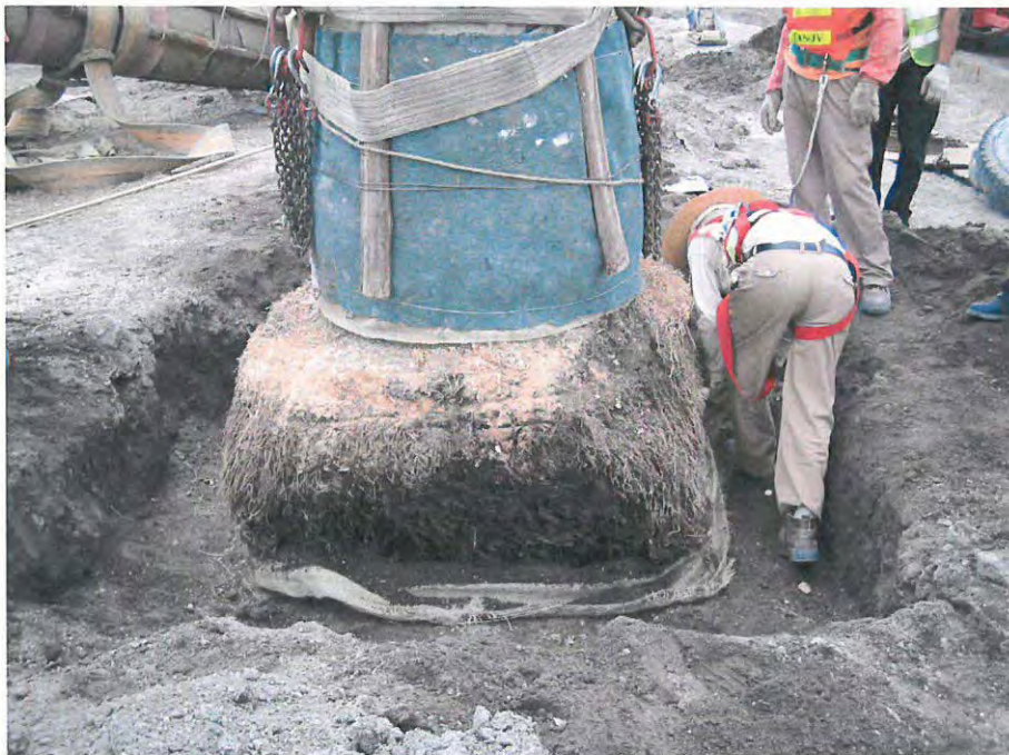
Replanting removal of root ball packing and backfilling with soil mix
