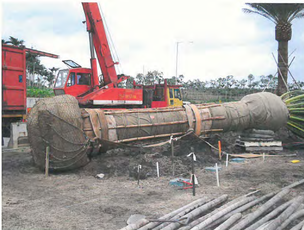
Root ball and wrapping to palm for protection during relocation and replanting
