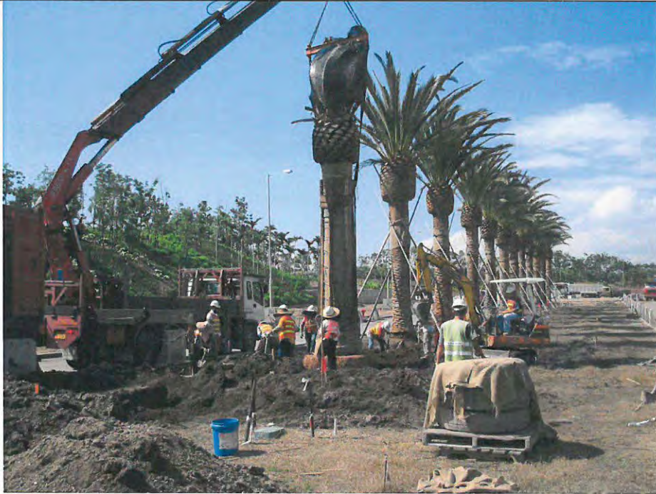
Method to lift and replant Elaeis guineensis 油棕 palms using a Crane Truck on EVA within Victoria Park.
